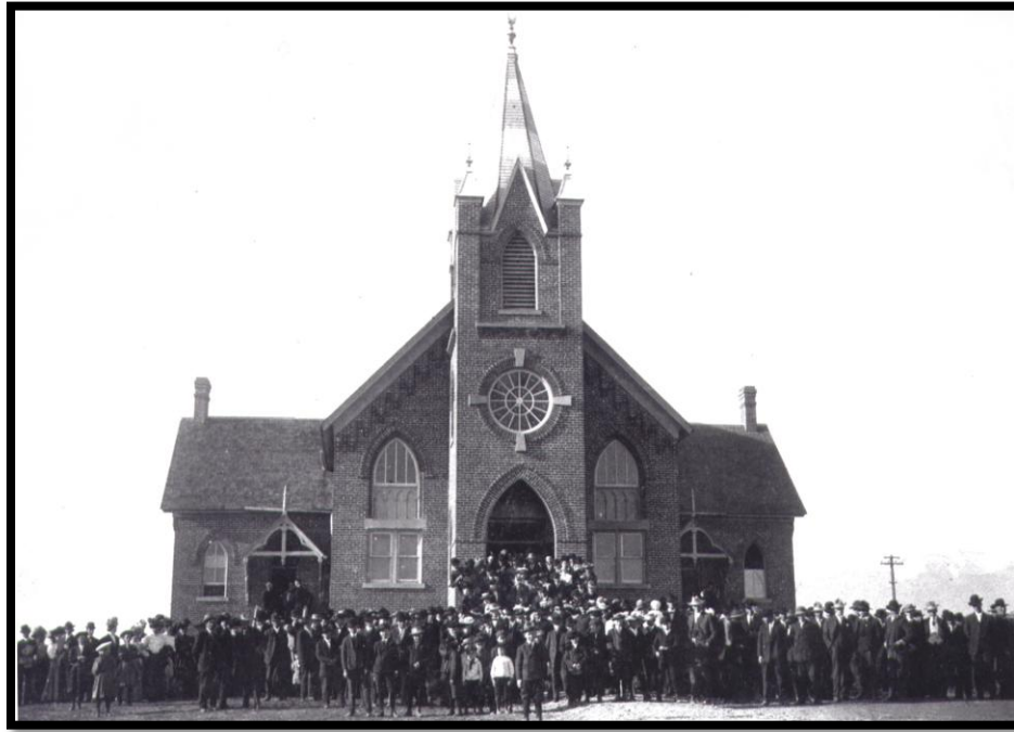
The members of the Layton Ward pose proudly in front of their new red brick chapel in 1908.
